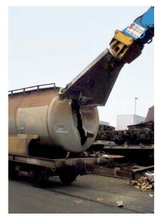
Heavy machinery for scrapping tank cars: scrap shears in use.
