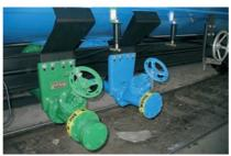
Drain valves: gas phase (green) and liquid phase (blue).
