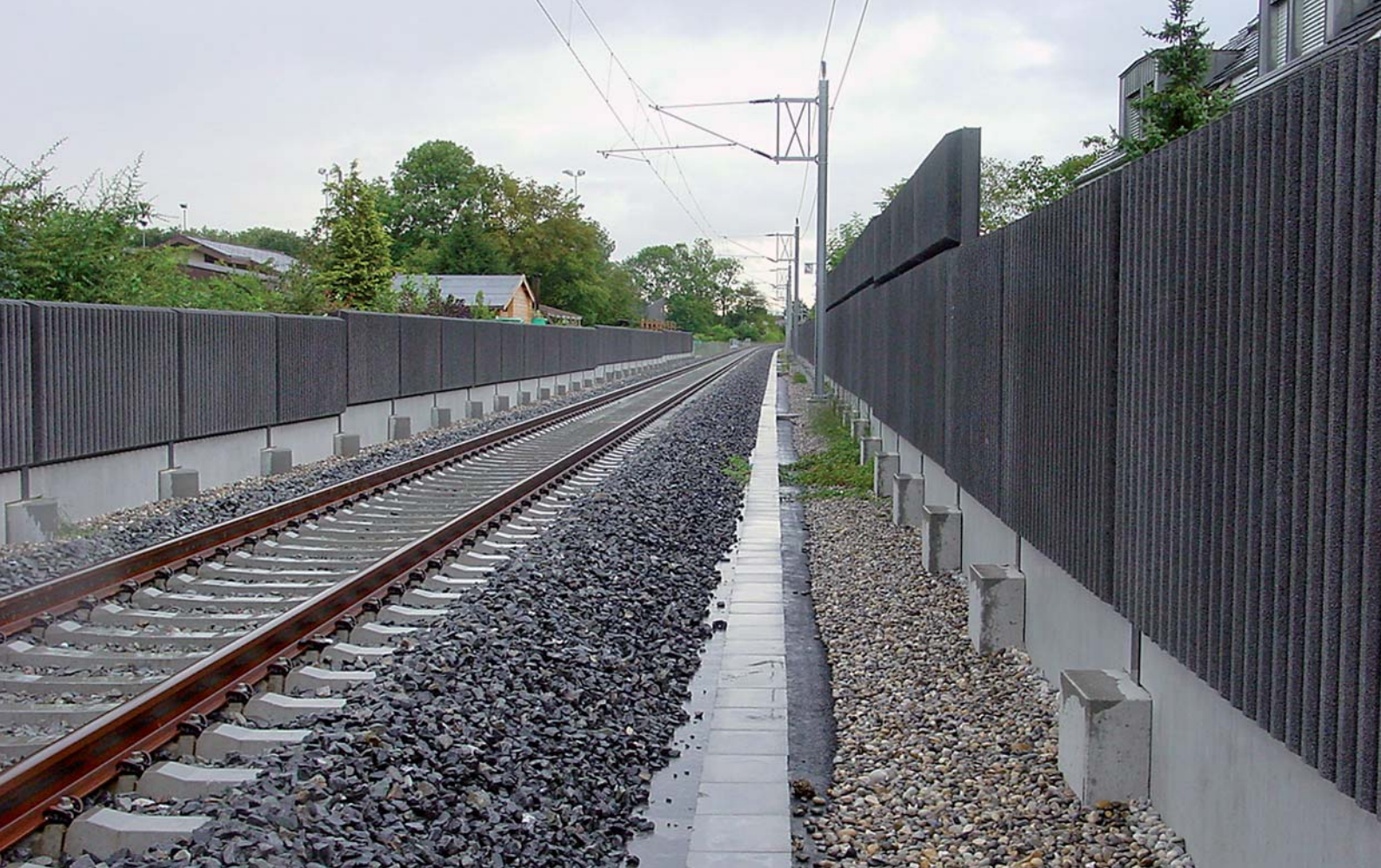
Noise-protection walls – expensive, but effective in reduction of sound emissions.
