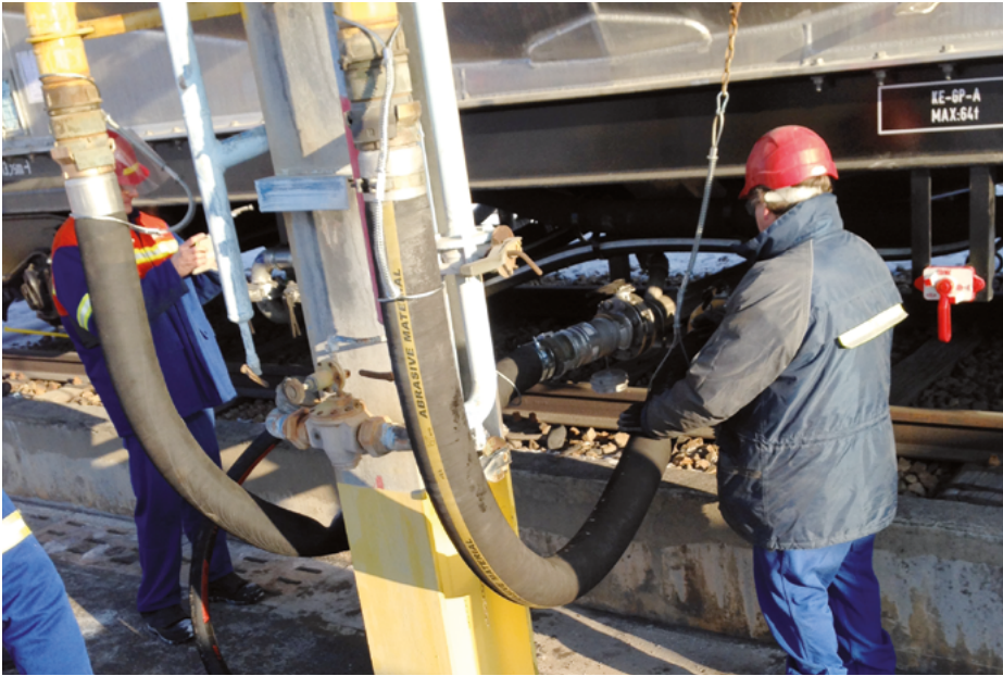
Test discharge, measuring the time taken to empty the tank
